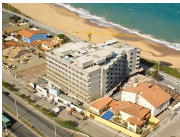
Figura 38: Macaé Palace Residence - 2005
