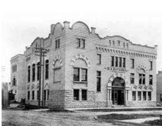
Figura 14: Salvation Army Citadel , em 1903. Fonte: Centre for Indigenous Environmental Resources.
