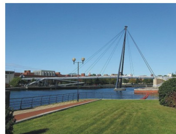
Teesquay Millennium Footbridge, Stockton-on-Tees, Inglaterra Foto: John Yeadon, 2009.
