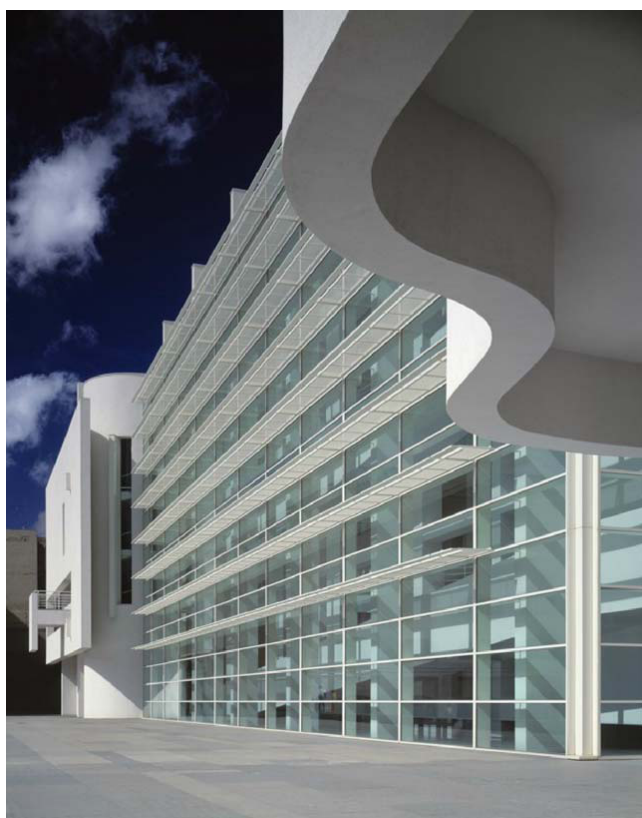
Figura 21 – MACBA – Vista externa Fonte: < http://www.richardmeier.com/www/#/project/s/architecture/type/institutional/1/123/0/ >. Acesso em: 18 nov. 2012.
