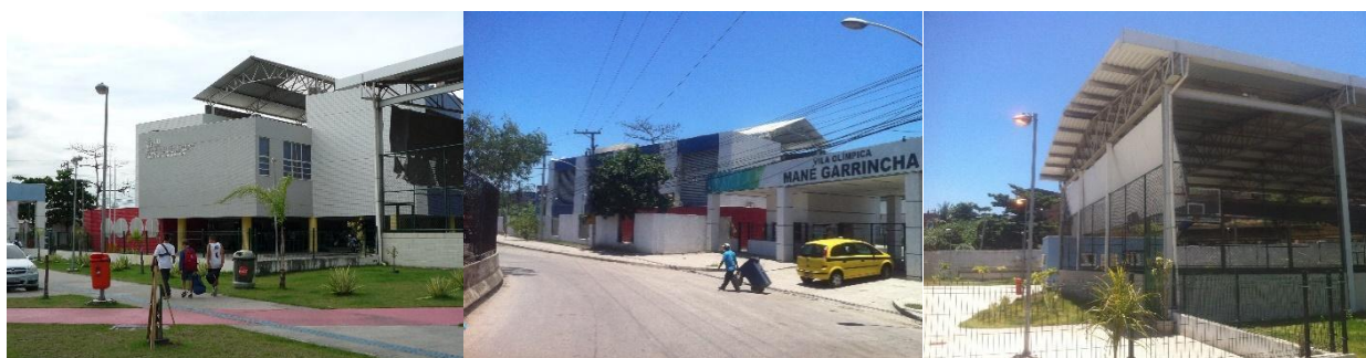
(a) Fachada principal GEO Caju
