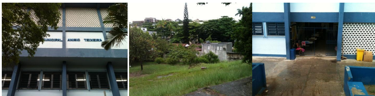
(a) Fachada principal
