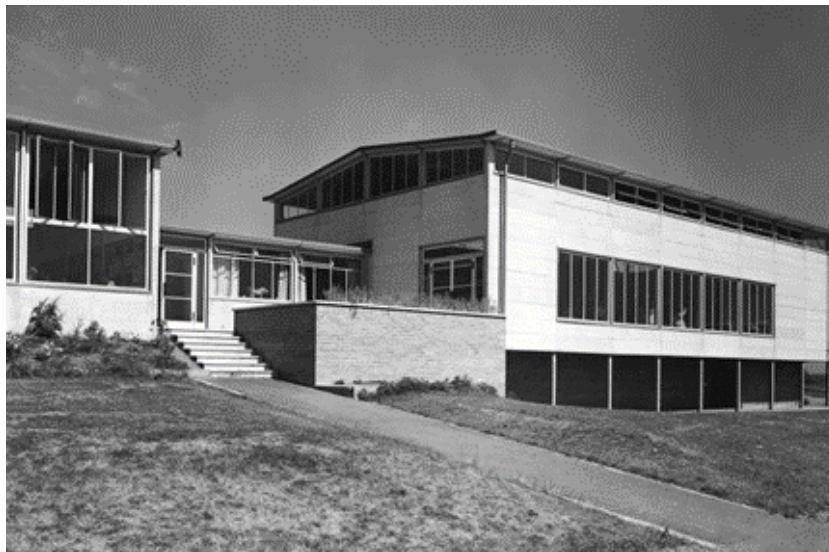
Figura 31 – Essendon Primary School , Hertfordshire, Inglaterra (1948). Disponível em: www.architecture.com/image-library/ribapix/image-information/poster/essendon-primary-school-hertfordshire-the-main-entrance-with-the-hall-on-the-right/posterid/RIBA44177.html .
