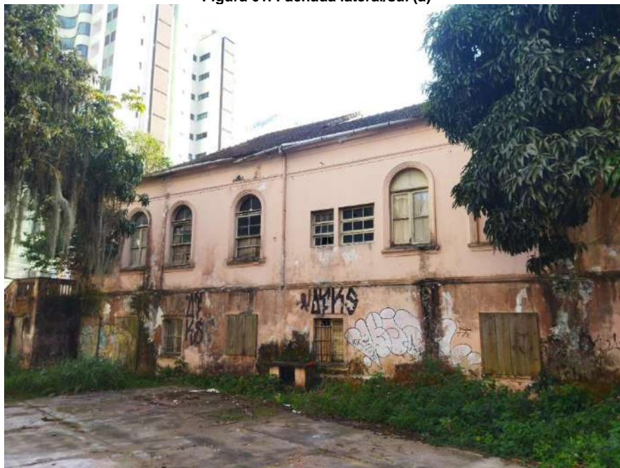
Figura 62. Fachada lateral/sul (b)
